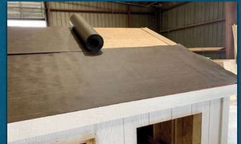
Tar Paper Under Roofing Only. Recommended for Shingle Roofs
