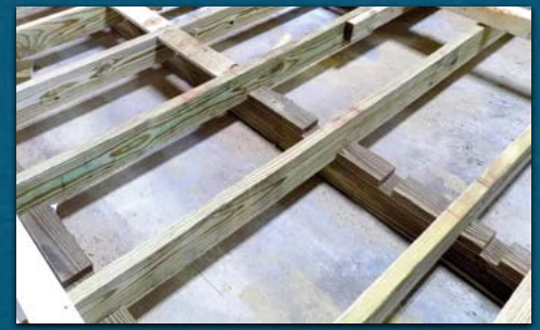
12" On-Center Floor Joists 16" OC is Standard
